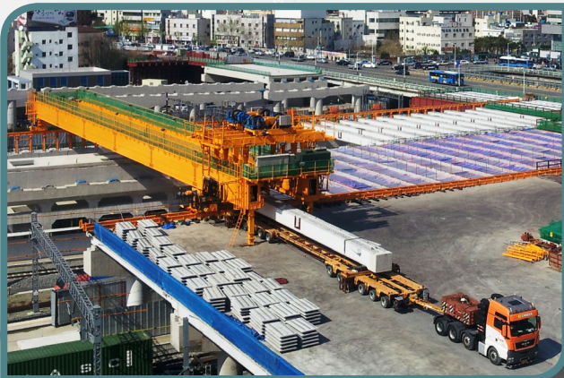
■ Edge Girder Erection Method
