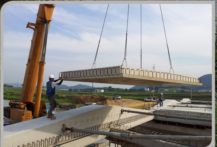
Erection of Precast Slab
