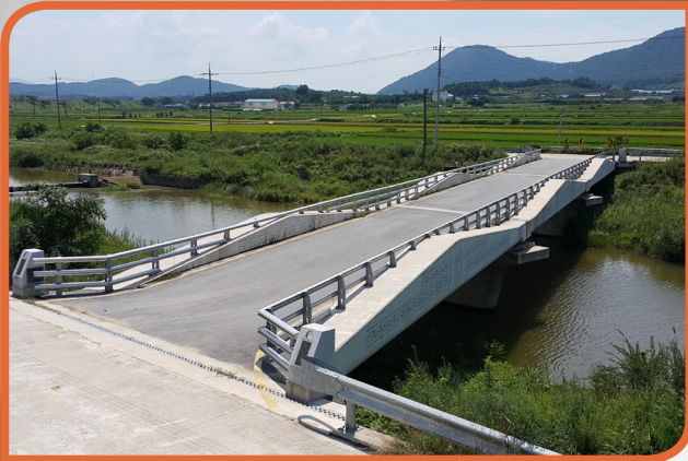
■ Precast Through PSC Girder
